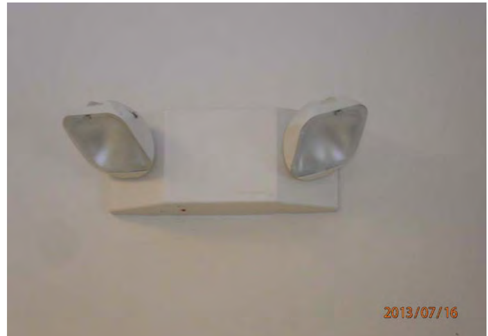
12. Community room inoperable auxiliary light fixture
