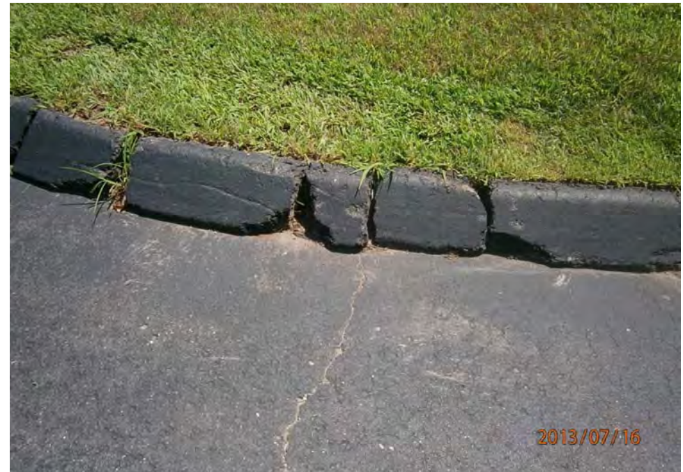
2. Damaged asphalt curbing
