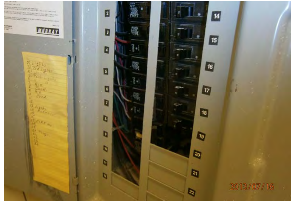
14. Community building circuit panel cover unfastened
