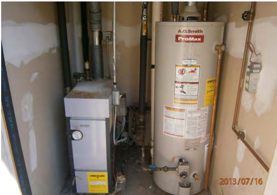
11. Community building boiler and DHW tank
