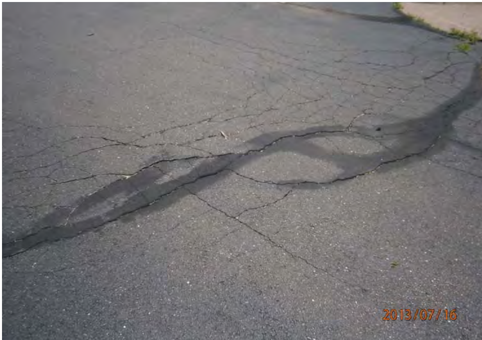
1. Asphalt roadway exhibits cracks
